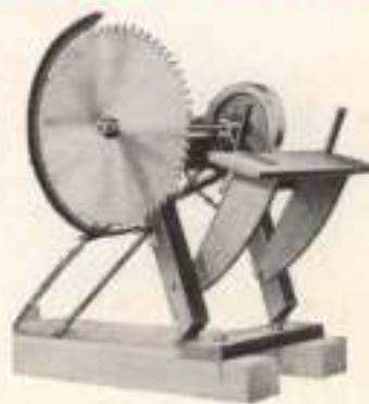
The tilting saw table
