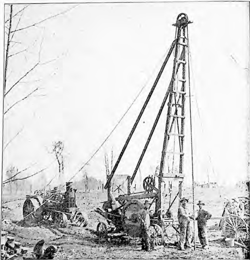
The Tractor not only furnishes abundant power for operating this machine but also will move it from place to place.
