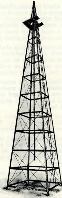
No. 1—50-ft. Tower, Girts 5 ft. apart. For 8 and 8½-ft. mills. 2 inch by 2 inch angle corner post
